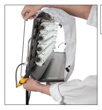
Remove Louver. Stretch two elastic cords around fixture. Take up slack on both elastic cords.
